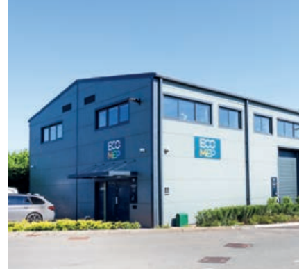
ABOVE: The new ECO MEP premises TOP LEFT: CES provided lifecycle information about its products BELOW: ECO MEP's state-of-art HVAC
