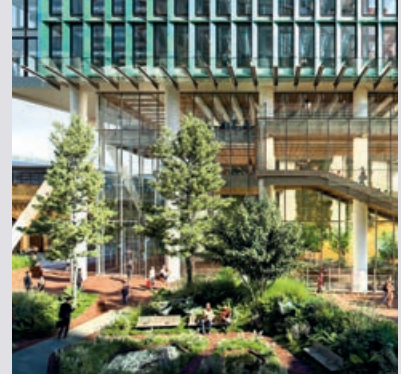
ABOVE: Edge will use smart tech throughout the new building in London
